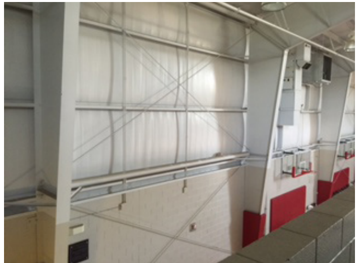
Typical Interior Wall Construction
